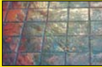
6" Grouted Slate Tile
